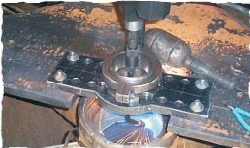
Repair on Stainless Steel Pump Housing Using Boretech Welder
